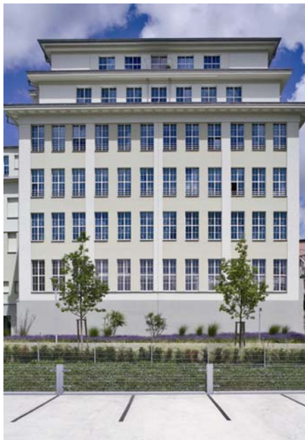
Hans-Sachs building: The GlassWin system from profine GmbH for the more than 1,000 new windows in the block allows an exact reproduction of the historical façade appearance.
